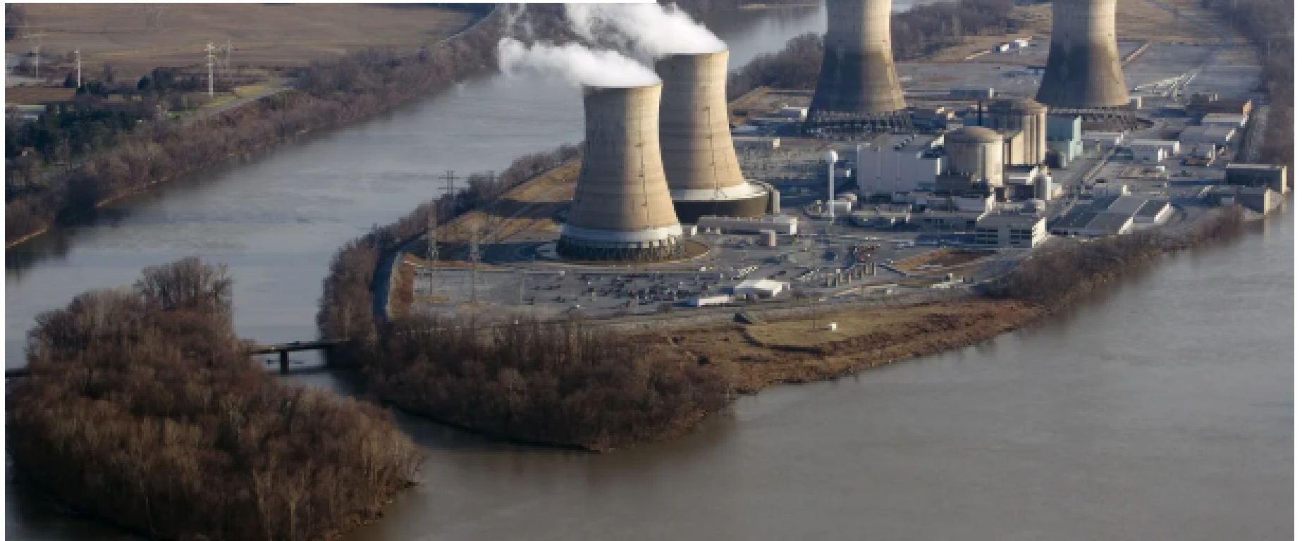
Cooling towers at the Three Mile Island nuclear power plant in Middletown, Pennsylvania. Photographer: Andrew Harrer/Bloomberg
